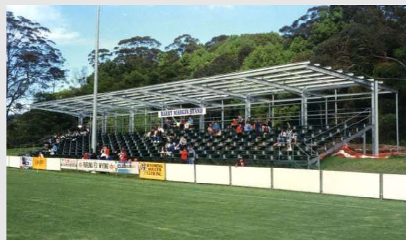
The Barry Margin Stand under construction.
